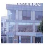
A full-glass curtain wall is another type of non-frame curtain wall where glass panels are connected with each other and eventually connected to the main building through peripheral supporting structures.
